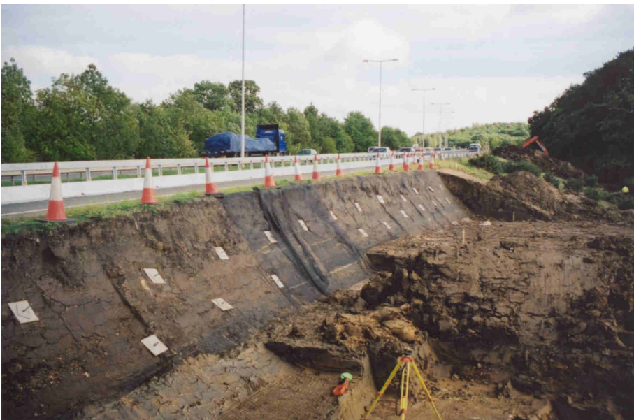
MR1 Duckbill anchors securing the A2 embankment at Boughton near Canterbury.
