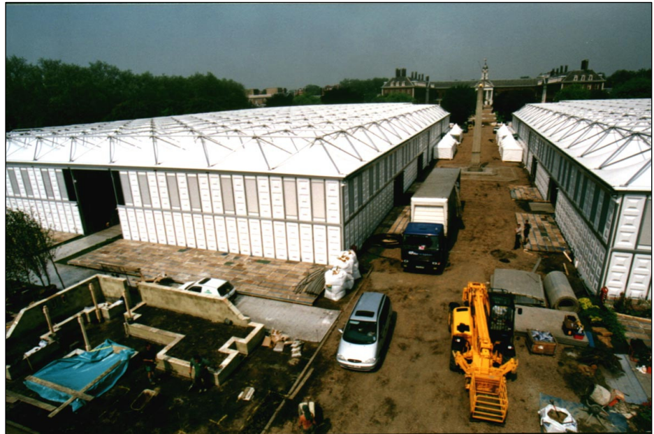
The two large temporary structures secured by Duckbill Stingray anchors
