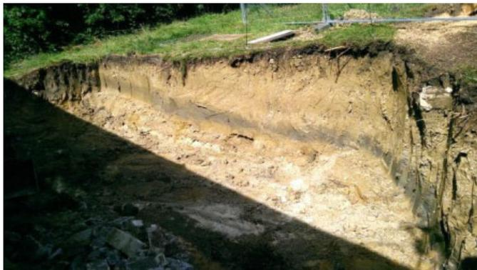
system such as gabion baskets. The gabion baskets although appealing for a gravity retaining system, could not achieve the required resistance capacity to hold the large cuttings from moving. SR Architects decided to discuss the use of our mechanical anchoring system to help with the design process to replace the counterfort walls.
