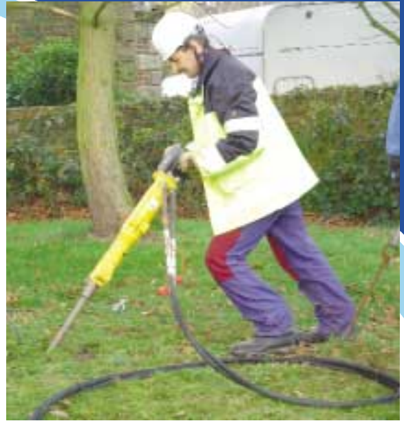
Driving the anchor
