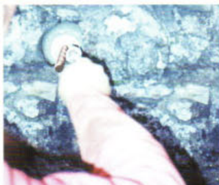
Fully inflate sock by injecting flowable grout and leave to cure
