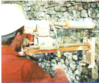
Remove stone or brick and core drill clearance hole
