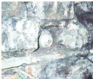
Replace stone, brick or cored material and make good
