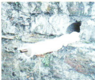
Insert grouted sock anchor of specified length
