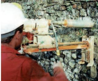
Remove stone or brick and core drill clearance hole
