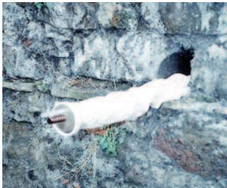
Insert grouted sock anchor of specified length
