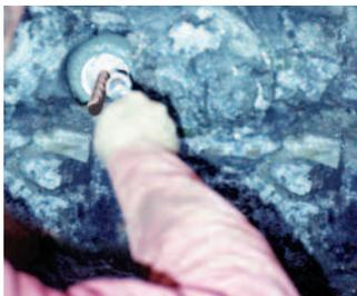
Fully inflate sock by injecting flowable grout and leave to cure
